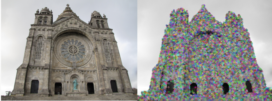
Figure 3: Example of keypoints extracted on Santa Luzia Church in Viana do Castelo (at the right).
